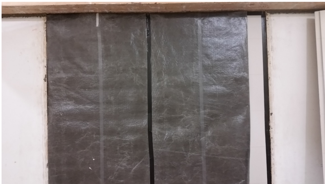
Figure 6 – Product under test partially installed, as viewed from source room
