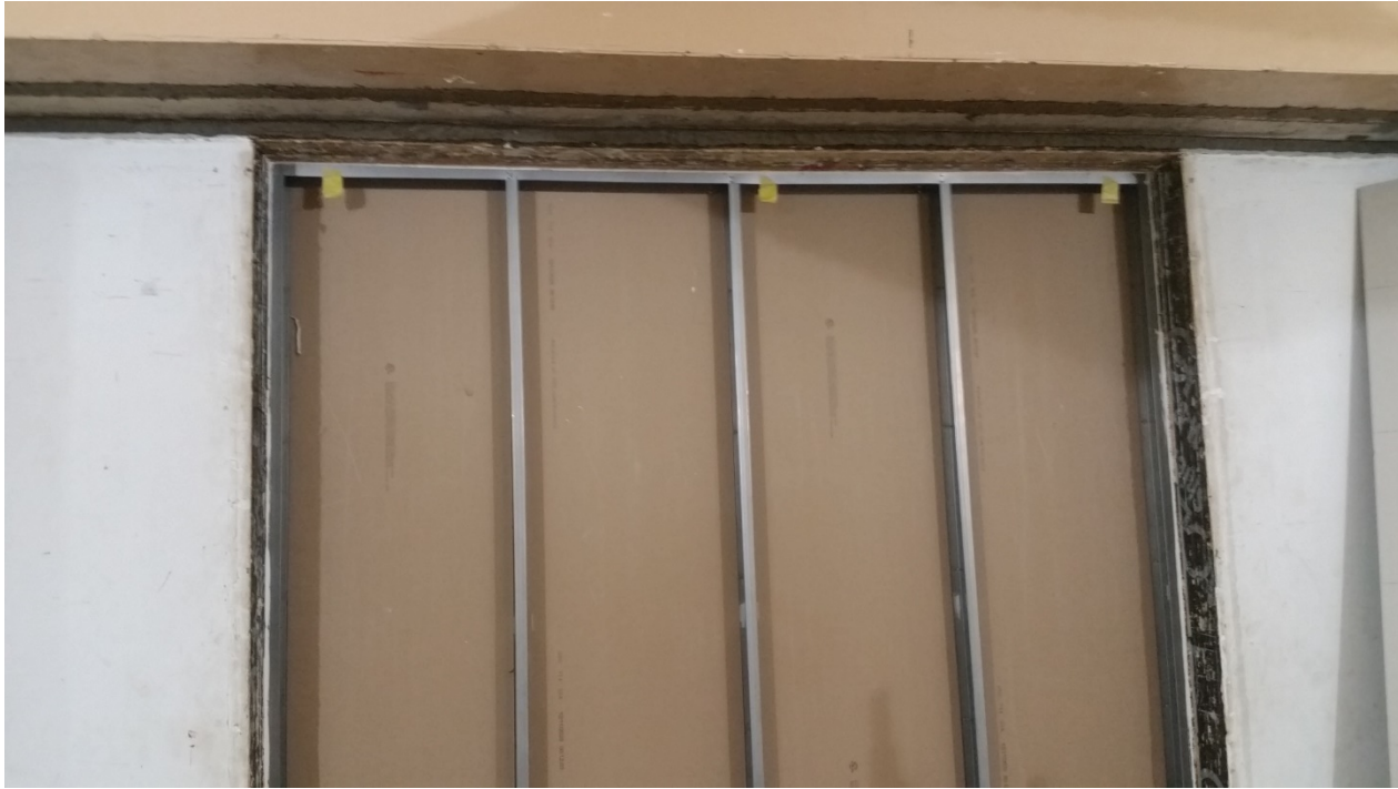
Figure 3 – Installation and sealing of steel framing members
