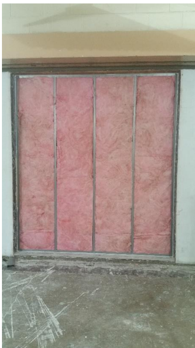
Figure 2 – Framing members and cavity insulation installed
