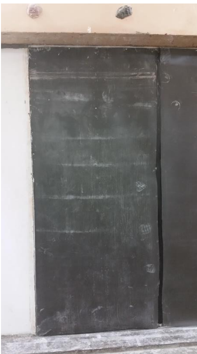
Figure 4 – Mass loaded vinyl layer installed
