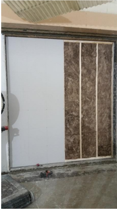
Figure 3 – Stud cavity insulation installed, receive side gypsum board partially installed
