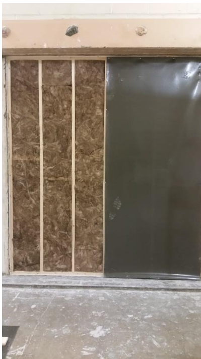
Figure 4 – dB-3 Lite layer partially installed, as viewed from source room
