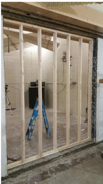
Figure 2 – Framing members installed in test opening
